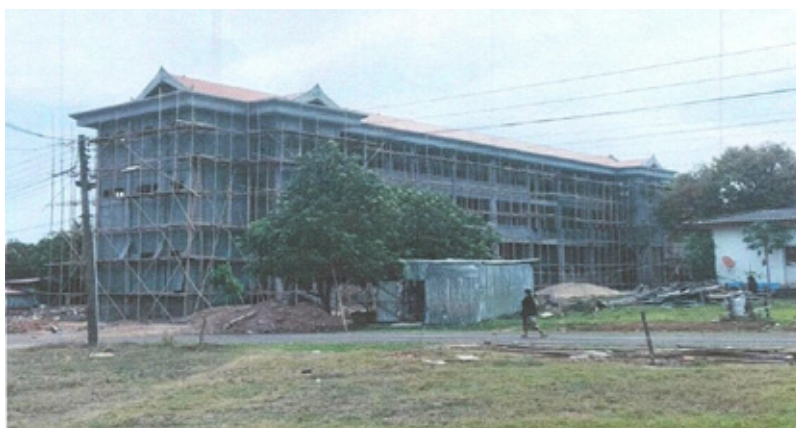
The three-storey classroom block at the grassroots health protection center of Salavan province, funded by Binh Dinh Province, having been promptly completed
