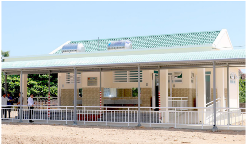
No. 2 primary school's toilet - Dap Da ward, An Nhon town, Cooperation project between Binh Dinh province and two French unions SEAFF/SFL
