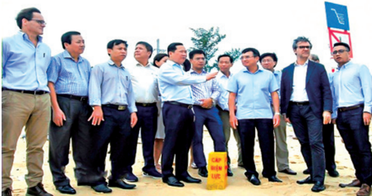
Mr. Nguyen Phi Long, Vice Chairman of the Provincial People's Committee (fifth from the left) and the mission members at the cable construction site (Photo Credit: NX)
