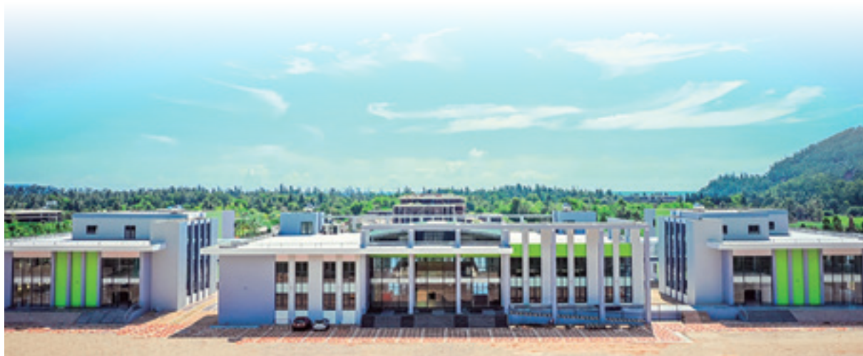
Overview of TMA Innovation Park (Photo credit: NX)
